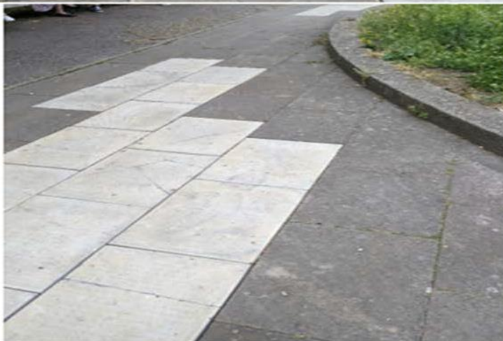
Figure 26: Paving and bins improvements at St. Paul's
